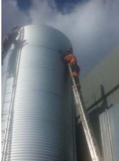
The steel panels of the tank are coated with a Aluzinc layer on both sides. The corrugated steel sheet is continuously hot dipped in a formulation of Aluminium (55%) Zinc (43.5%) and Silicon (1.5%). The aluminium components of the coating provide a tough physical barrier between the extreme atmospheric conditions and the inner core steel. Aluzinc has inherent sacrificial properties and corrodes first before the mild steel corrodes.
