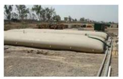
Aviation, commercial, transport, Defence Forces, UN Aid and industrial application for Rapid deployment of any liquid storage are just some of the possibilities. The application and content for the Fuel bladders dictates the use of a bunded berm liner and, made from PVC or Polyurethane material, or optional inflatable Berm liner for secondary containment. As pillow tanks operate in a vacuum, what you put into a bladder is what you get out, no dust, air or light exposure to your product.
